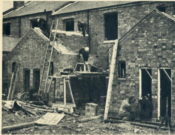
Building Repair after the Blitz
